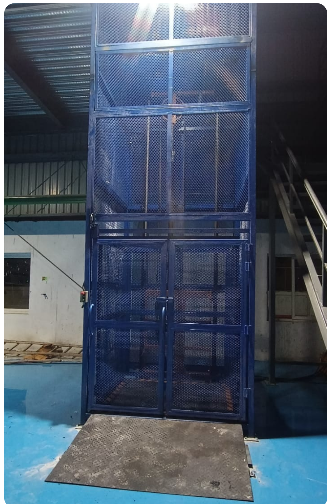
Double Mast (Goods Lift) With Wiremesh Structure
