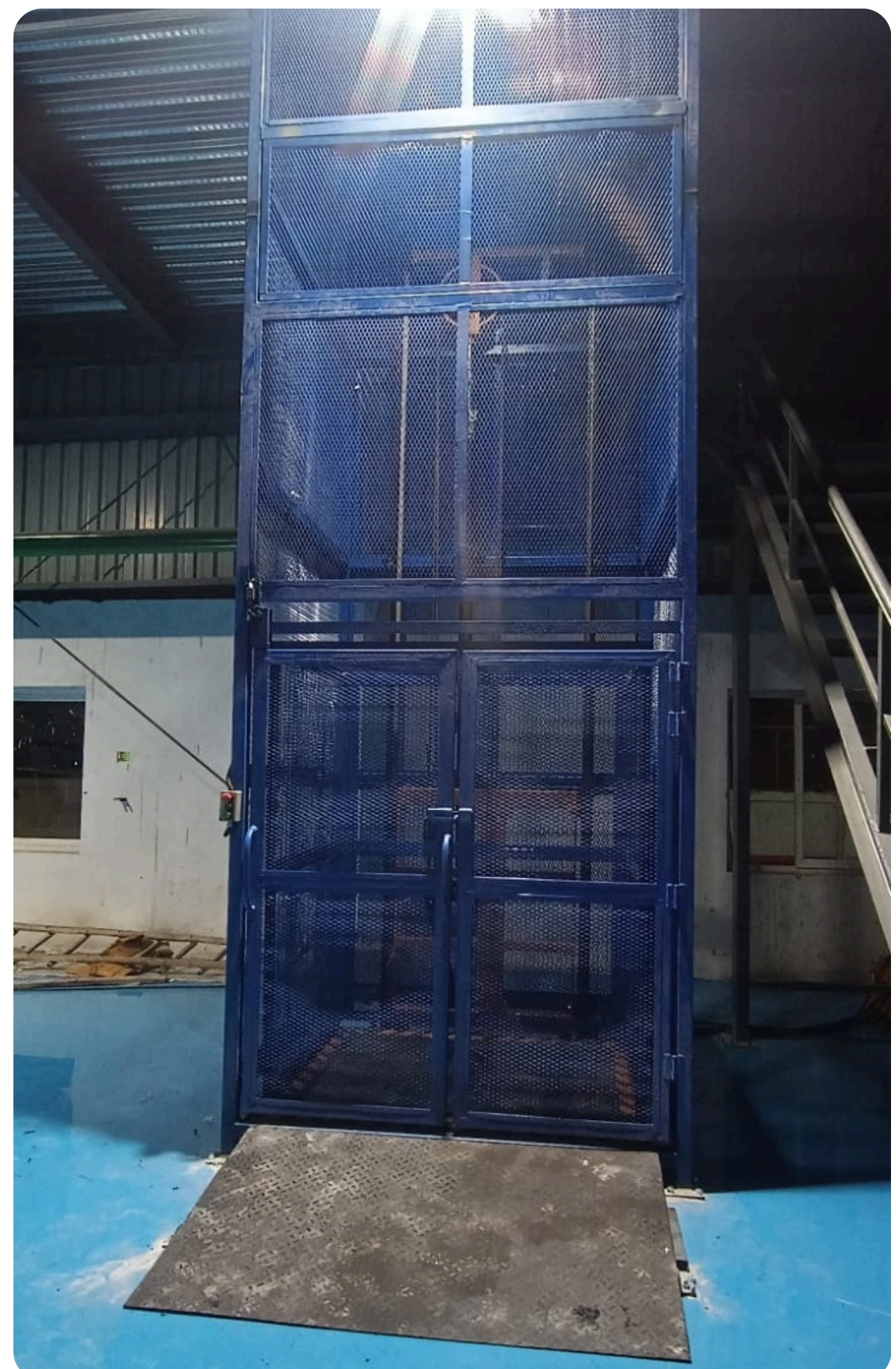
Double Mast (Goods Lift) With Wiremesh Structure
